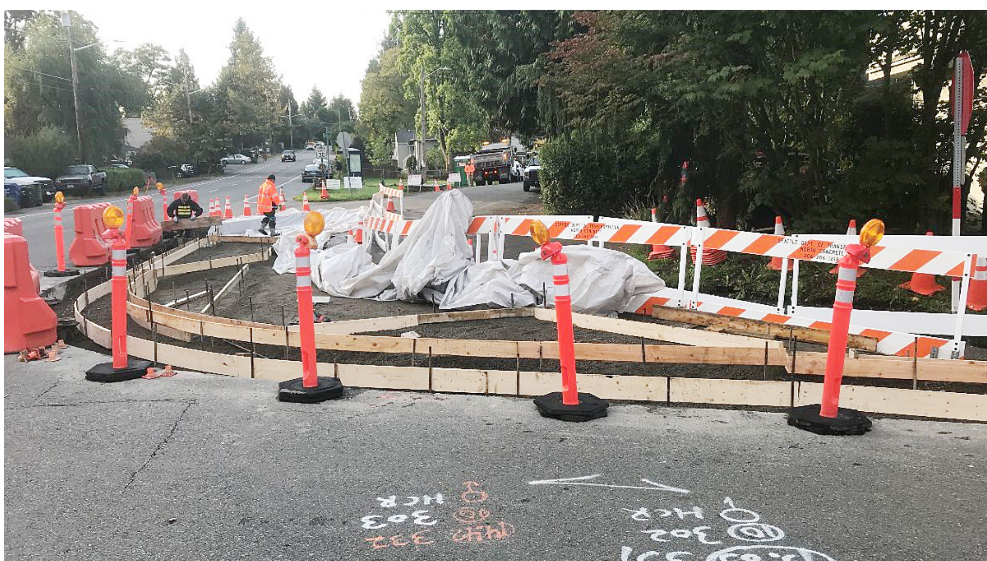
Curb bulb replacement before and after on Sand Point Way NE and NE 125th St
